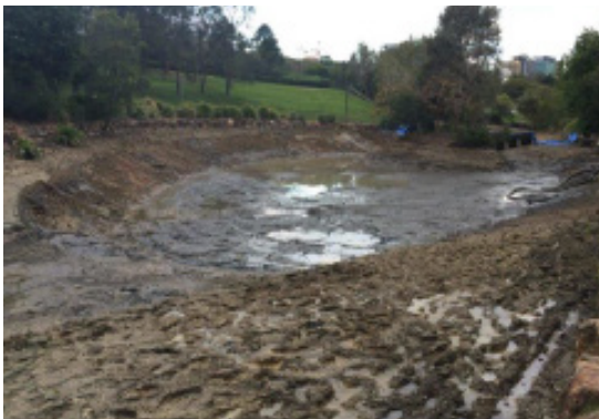
Dewatered and desilted Q3 and Q4
