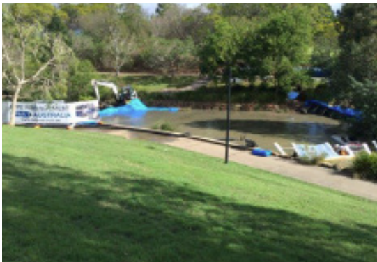
Q2 with installation of B2
