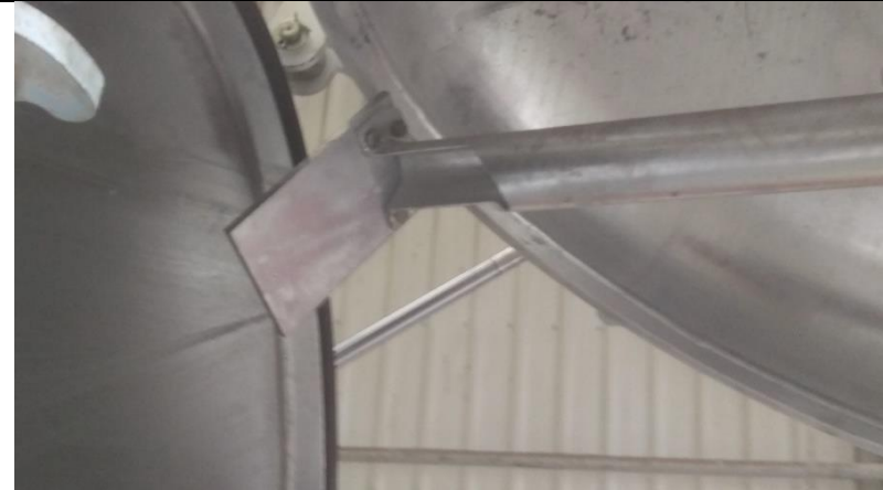
Deflection plate installed inside tank distribute materials evenly within the tank
