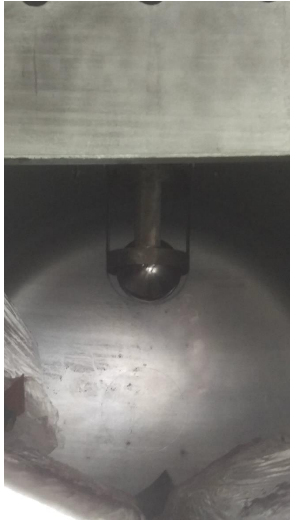
Rubber ball seat fitted which is the primary shut off when the tank is full. Inspection fortnightly by competent person
